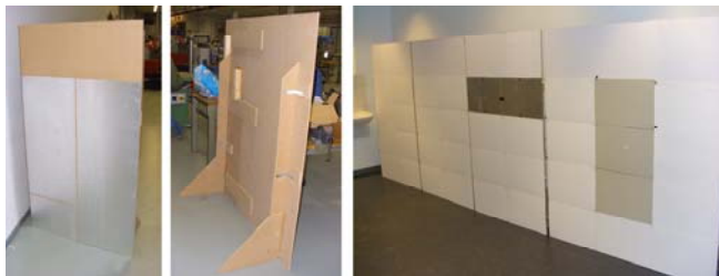
Figure 7. Wall construction with the aluminium foil and panels
